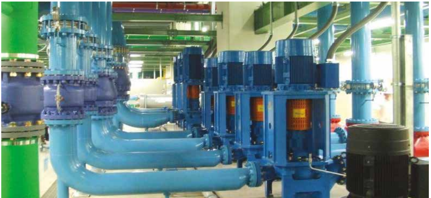
This ITT Goulds customer saved space as well as foundation and baseplates costs with seven Model 3910s. Many applications benefit from the inline piping as well.
