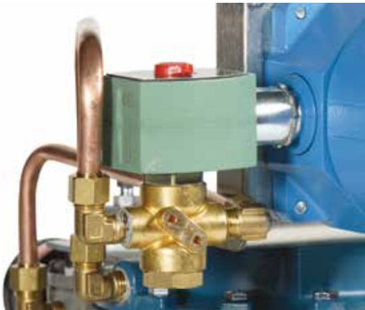
Asco Solenoid Valve
