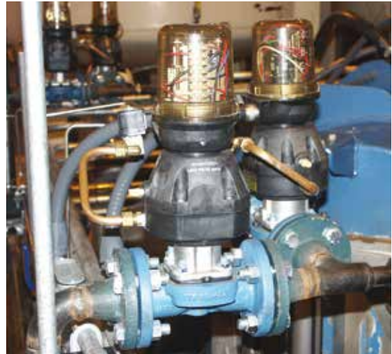
Dia-Flo® weir diaphragm valve with Advantage Actuator and SP2.0 switch pack.
