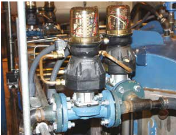
Weir Type Plastic Lined Valve with Advantage Actuator
