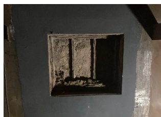
Anti-corrosion treatment of the inner wall of the fan flue duct
