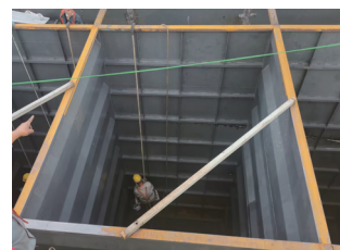
Anti-corrosion of the inner wall of the flue gas dust collector
