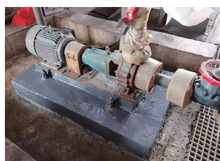
Anti-corrosion treatment of pump base
