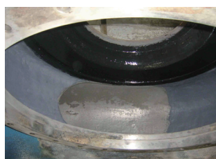
Pump casing repair
