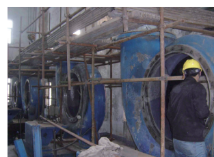
Corrosion prevention for the inner walls of corrosive tanks and vessels
