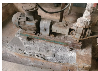
Anti-corrosion treatment of pump base
